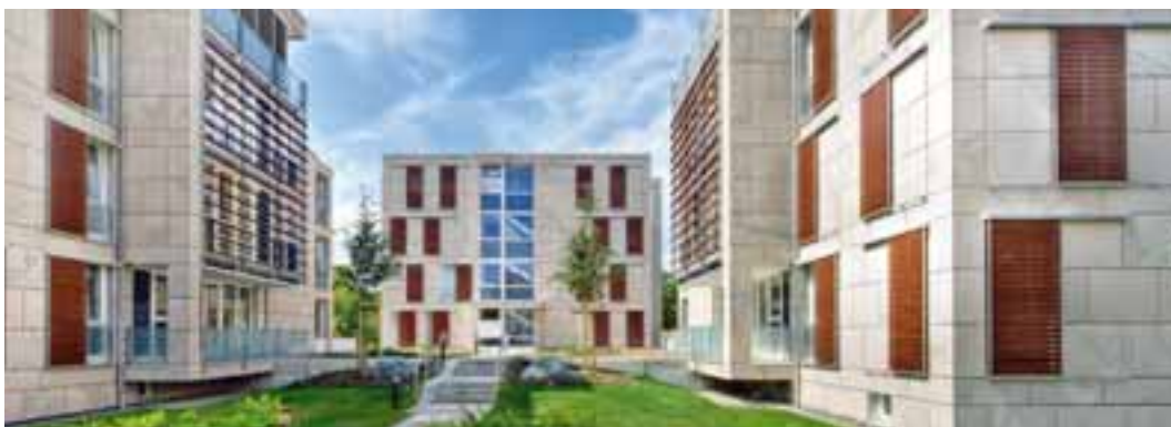
Town houses in Braunschweig with a ventilated rainscreen cladding system (StoVerotec Stone Massive with Sto-Sandstone Neubrunn)
