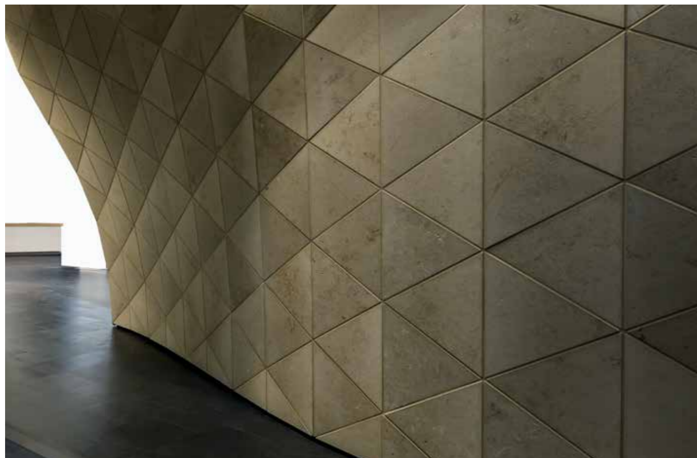
Sto messestand Bau 2015, DE-München; Arkitekt: FAT LAB, DE-Stuttgart, Foto: Martin Baitinger
