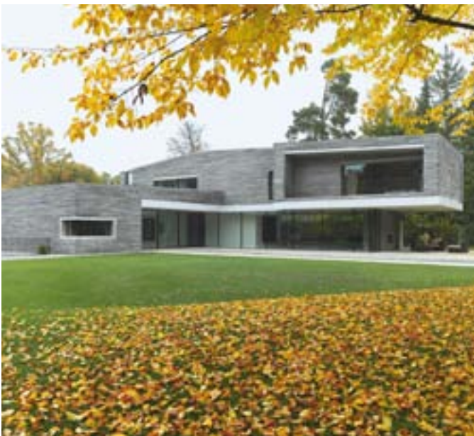
House M, constructed using a self-supporting natural stone facade
