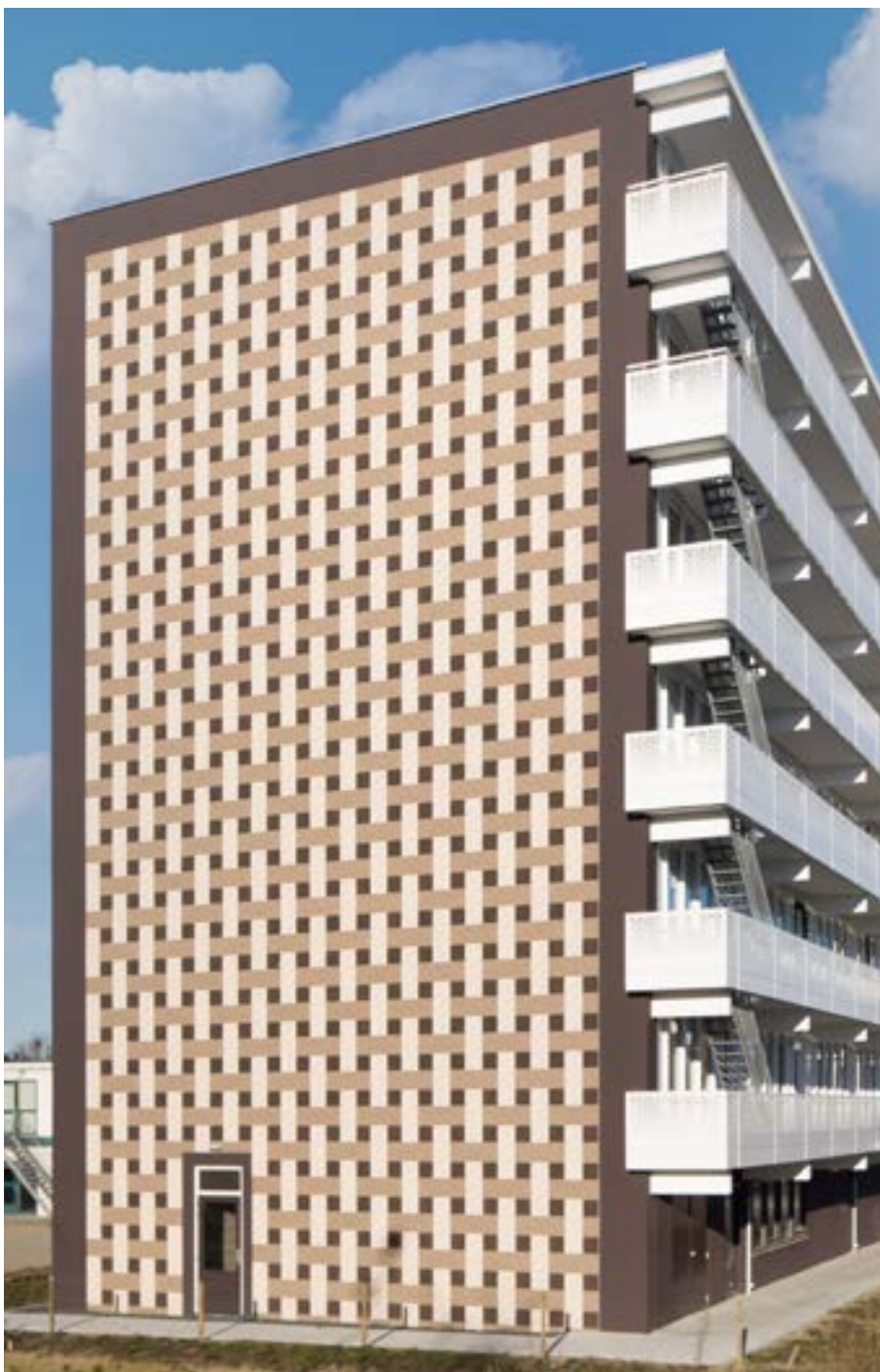
De Wever, Gennepe, NL Building owner: Mooiland Wonen, Grave, NL Design: 2.0 Architecten, Venlo, NL Execution: IJsselmonde VOF, Rotterdam, NL Sto expertise: StoTherm Classic®, StoCleyer B, StoEcoShape Photo: Bona Pictura, Cuijk, NL
